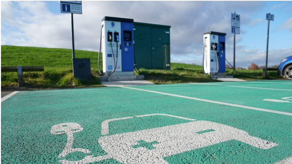
Figure 4. An electric vehicle charging point in the UK.
